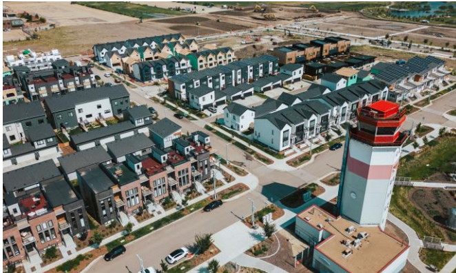
Ongoing land development and home construction
