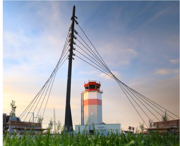
Control Tower before renovation
